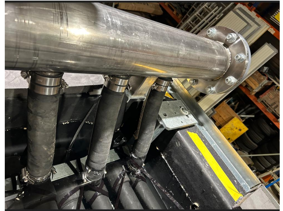
Glycol water Manifold & pipes to connect the exchangers
